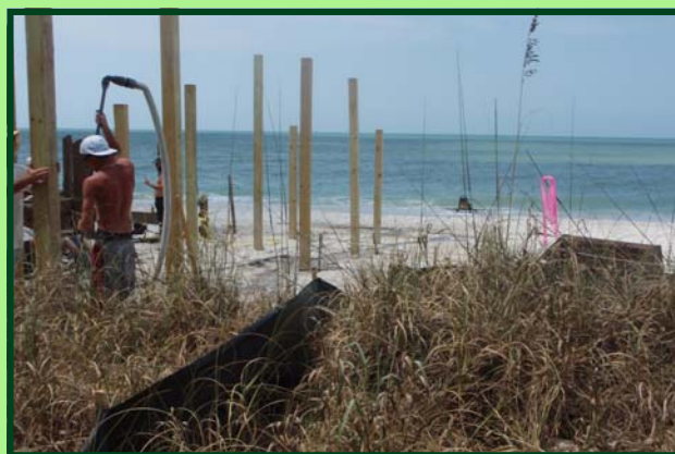
Below: Gopher tortoise burrow protected by silt fence during dune walkover pile installation.
