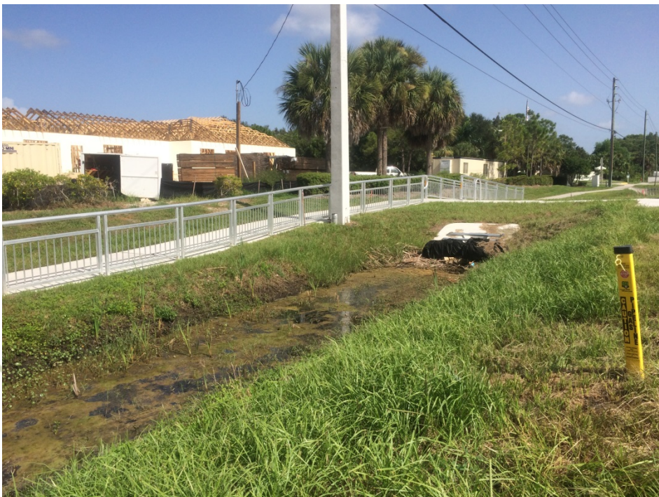
Picture 3: Bus Stop Improvements looking into site from South
