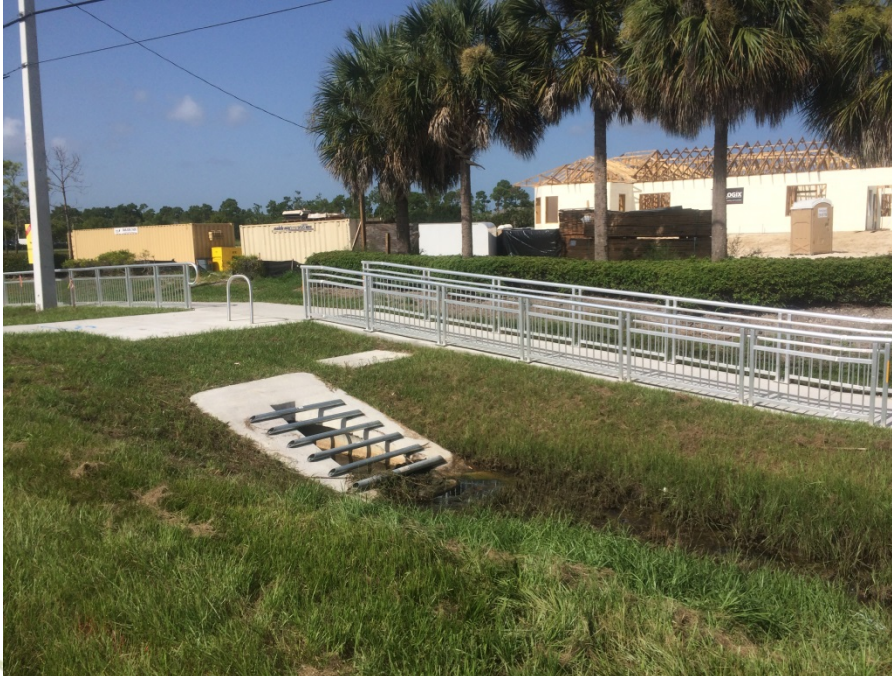
Picture 1: Bus Stop Improvements looking into site from North
