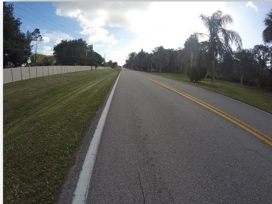
Figure 8 Longitudinal and Alligator Cracking in Wheel Path - Sandy Lane
