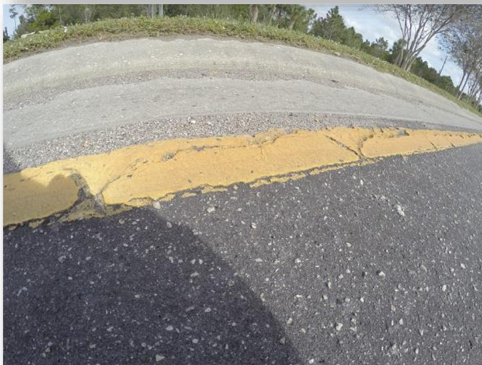
Figure 3: Severe Raveling & Road Not Flush with Curbing - Estero Parkway
