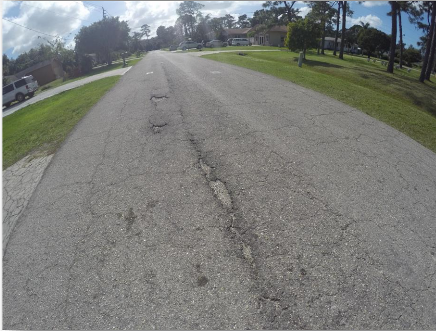
Figure 5: Potholes and Large Patches – Poinciana Avenue
