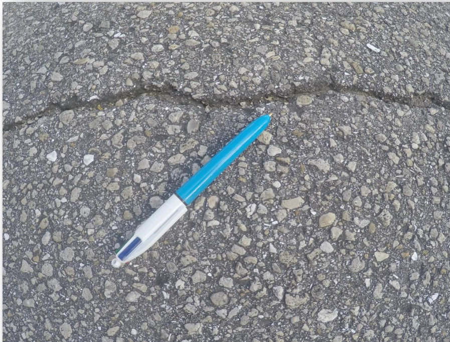
Figure 9: Type III Cracking Along Wheel Path – Sandy Lane
