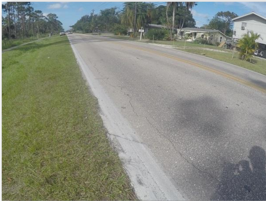
Figure 7: Alligator and Longitudinal Cracking in Wheel Path - Broadway Avenue
