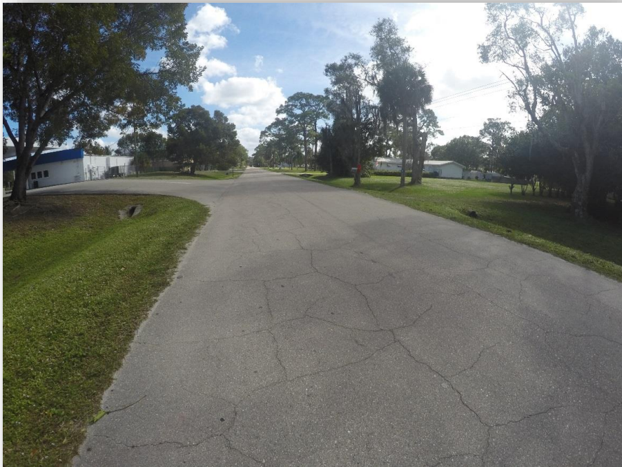
Figure 6: Type II Block Cracking Throughout – Trailside Drive
