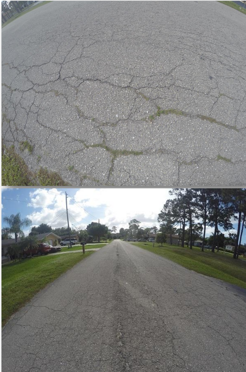
Figure 4: Exposed Base and Type III Alligator Cracking - Poinciana Avenue
