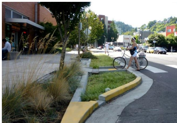
Left: Roadside bioswale intercepts stormwater from impervious surface (Source: National Association of City Transportation Officials (NACTO) text, "Urban Street Design Guide")
