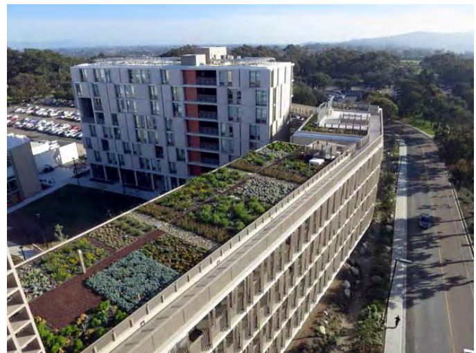
A green roof, like one shown in this example from San Diego, helps to reduce energy costs and stormwater runoff.
