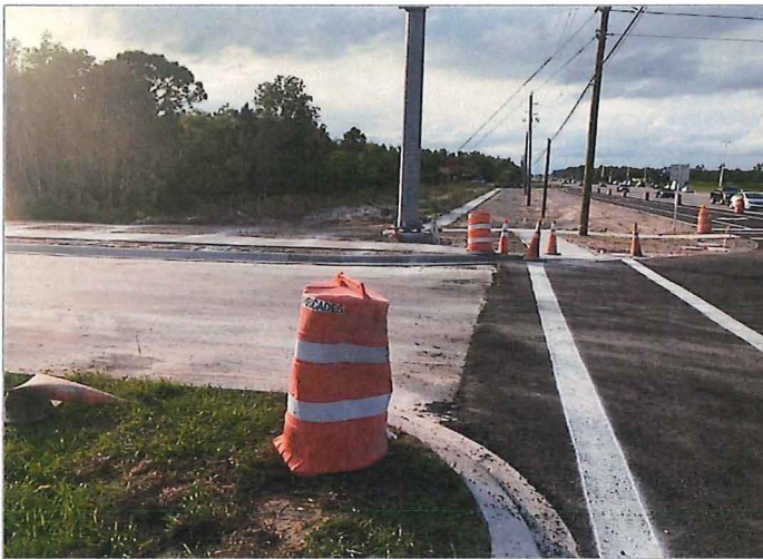
Figure 1 - Looking South from Terracap Way – turn lane and sidewalk improvements (April 4). The original right-of-way line was roughly along the telephone poles, the new is along the sidewalk. Notice the sidewalk jogs west due to donation
