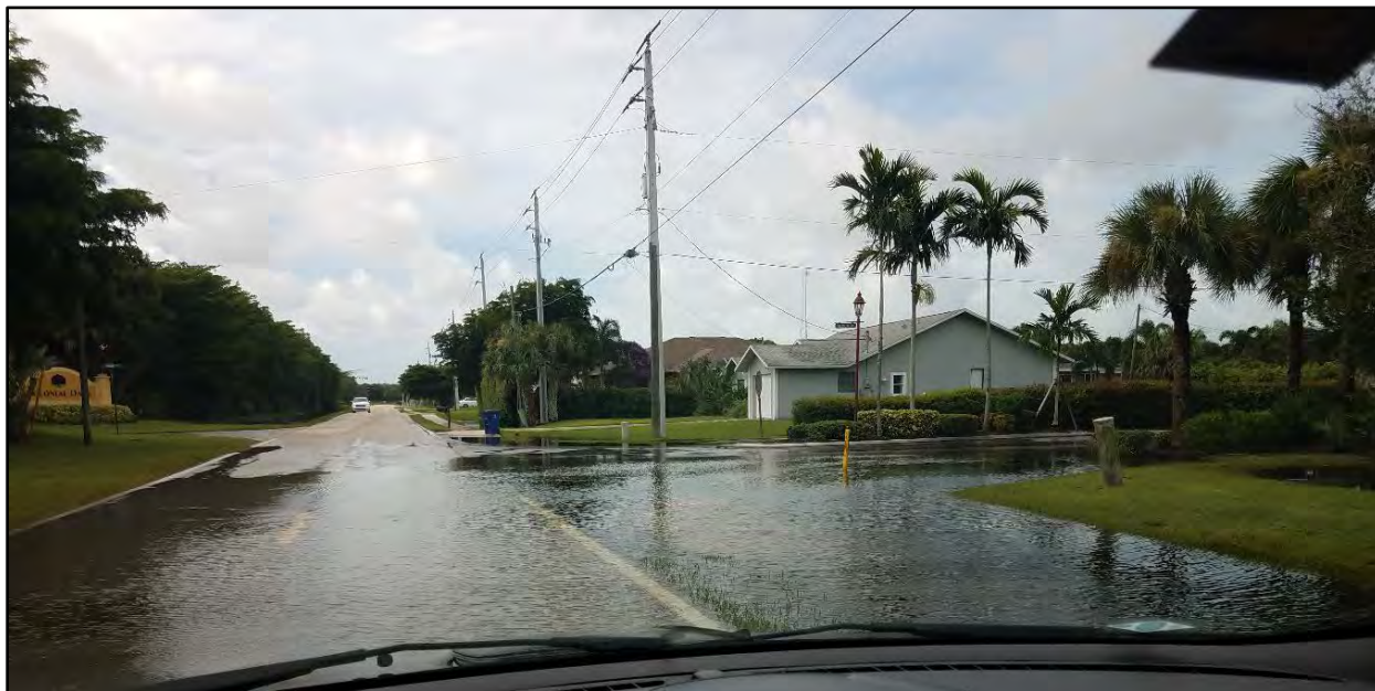
Figure 4-1: River Ranch Road and Block Lane, Looking South (August 28, 2017)
