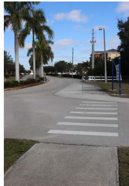
Sidewalk from Estero Community Park ends just outside the entrance to the park and does not connect to the surrounding community
