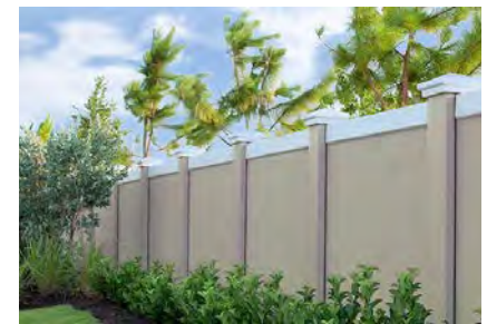
8' privacy wall of pre-cast, painted concrete along buffer (full buffer not shown)
