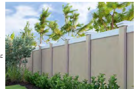
8' privacy wall of pre-cast, painted concrete on top of 4' berm along buffer (full buffer not shown)
