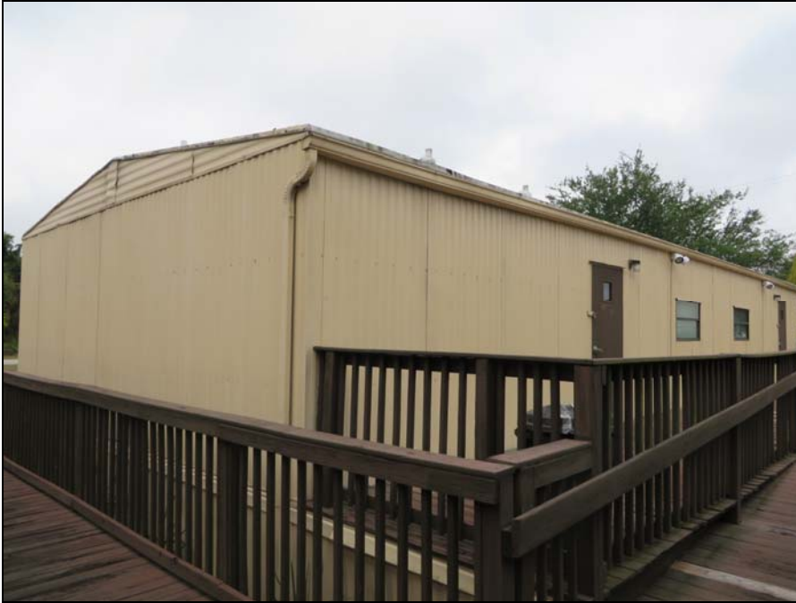
View: North Manufactured Building No. 3 (Fellowship Hall)
