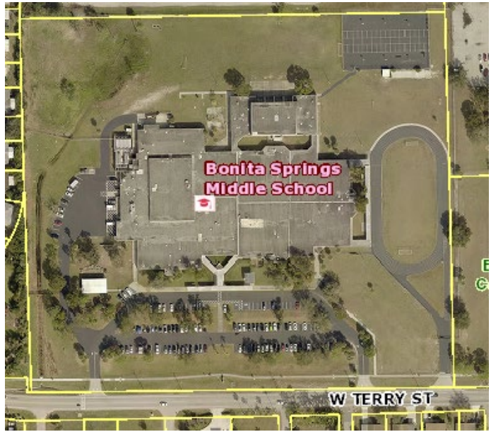
Figure 4: Aerial of Bonita Springs Middle School
