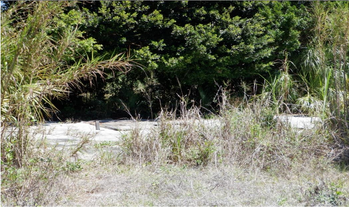
Photo 28: Structure 11 - 20911 Highlands Avenue 33928 – Concrete slab approximately 1,300 ft 2
