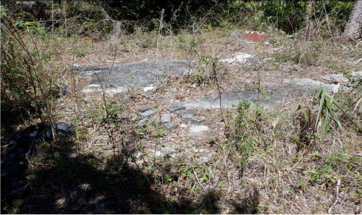
Photo 25: Structure 10 - Concrete slab approximately 500 ft 2
