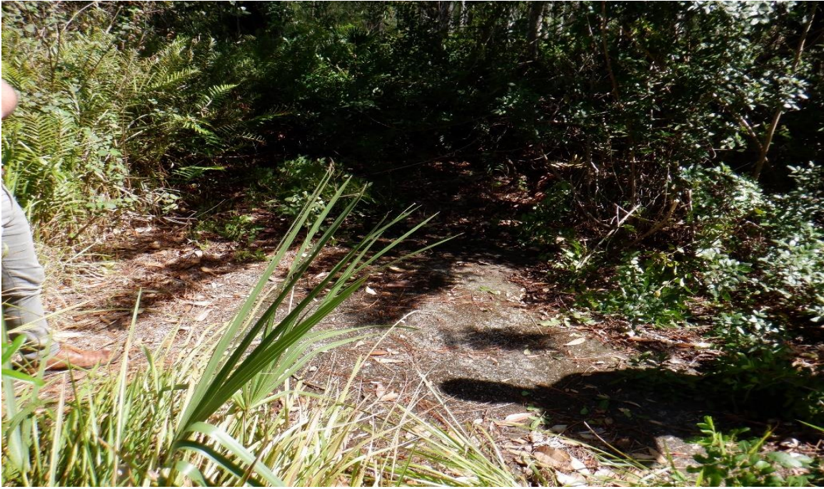
Photo 5: Structure 2 – Concrete slab approximately 100 ft 2
