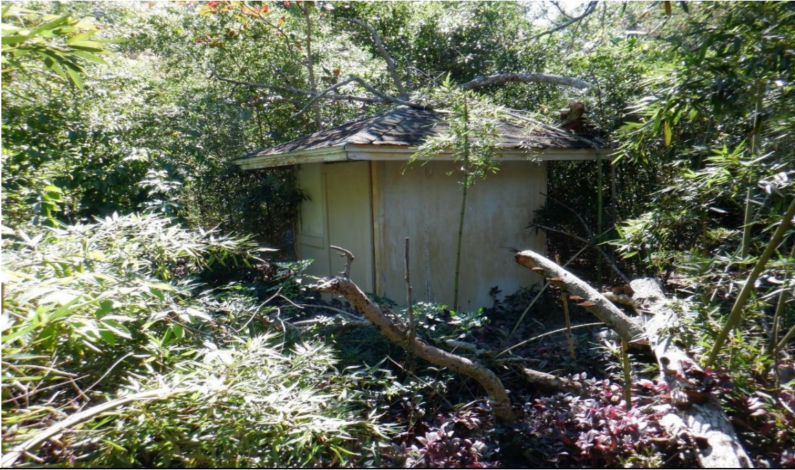
Photo 21: Structure 8 – Wood framed shed for well equipment.
