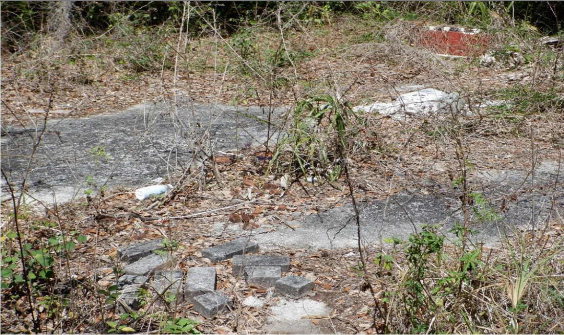
Photo 26: Structure 10 - Concrete slab approximately 500 ft 2
