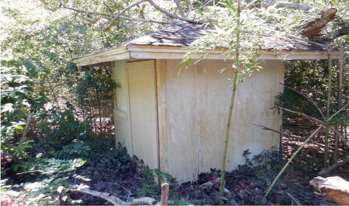
Photo 22: Structure 8 - Wood framed shed for well equipment.
