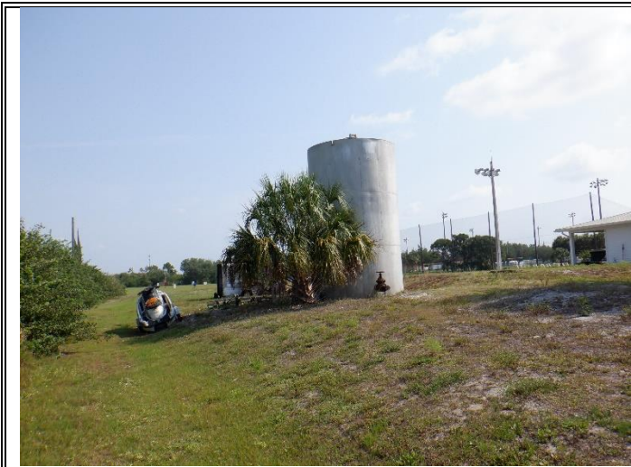
Photo 11: Water Tank on east adjacent property was observed.
