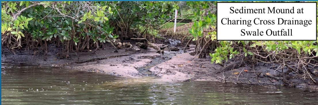
Sediment Mound at Charing Cross Drainage Swale Outfall
