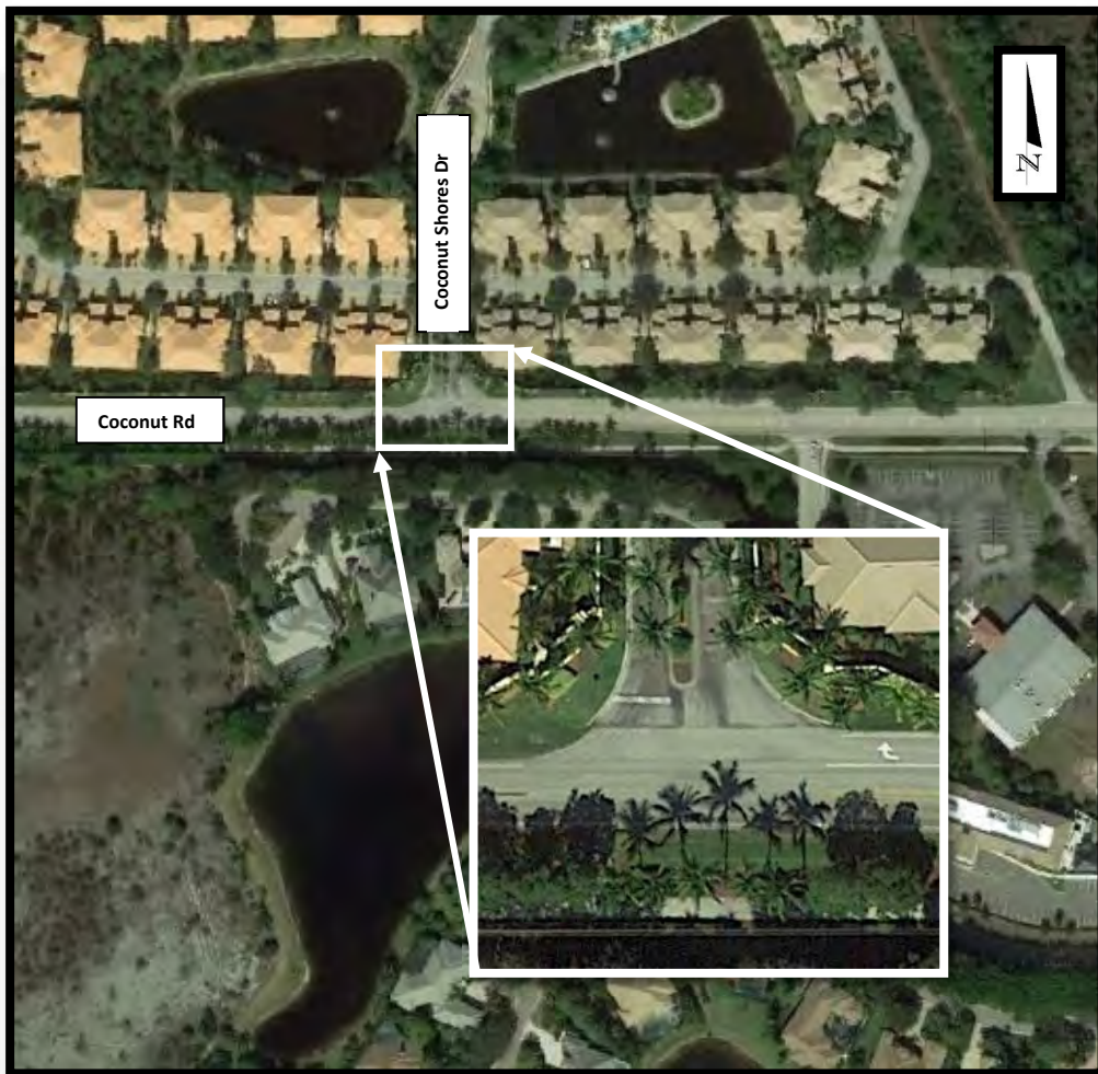
Figure 2-4 Existing Conditions - Location 4
