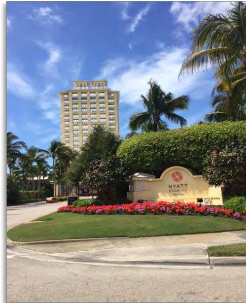
East-west portion of Coconut Road terminates at the Hyatt Hotel and the roads runs north-south for a short length (<500 ft) and then west for another 2,000 ft.
