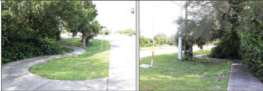
NORTHWEST CORNER - EXISTING CONDITIONS
