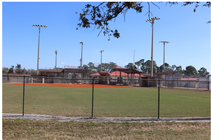
Three Oaks Community Park
