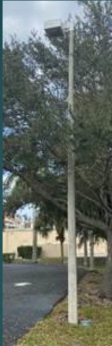
Existing Light Pole
