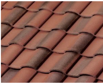
Roof with "Flashing"
