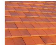
THE ROOF WILL BE A FLAT CONCRETE TILE WITH A TERRA COTTA COLOR
