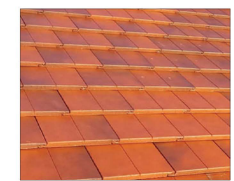
THE ROOF WILL BE A FLAT CONCRETE TILE WITH A TERRA COTTA COLOR
