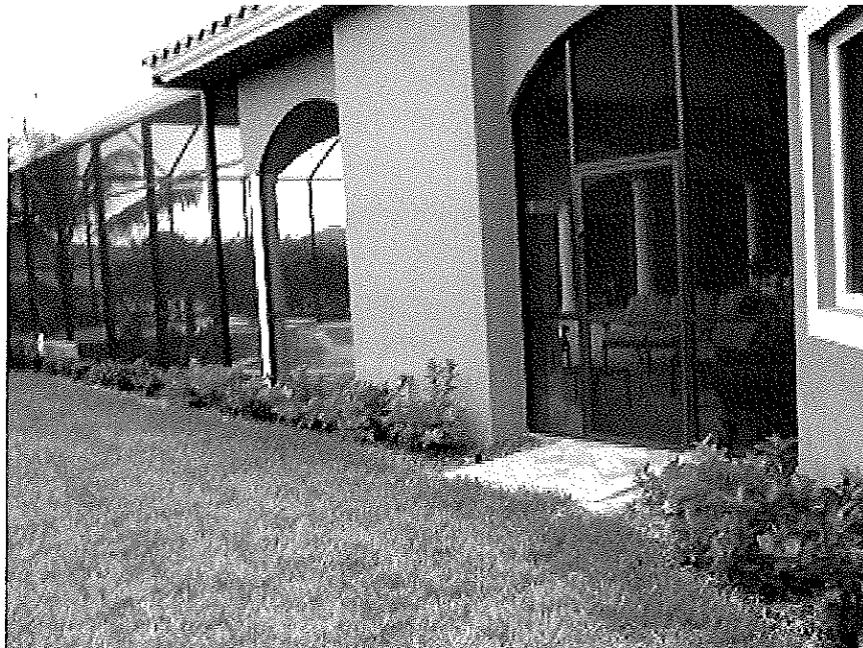
REAR VIEW (EAST) November 12, 2009
