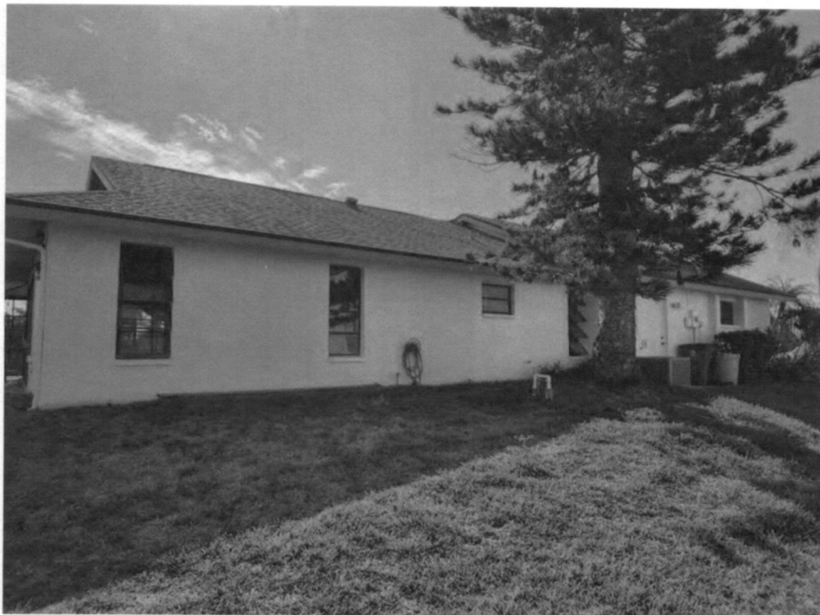
Photo Two Caption Photo Taken 12/12/2022 "Side View with A/C"
