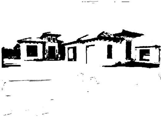
Front View Date Taken: 9/23/16
