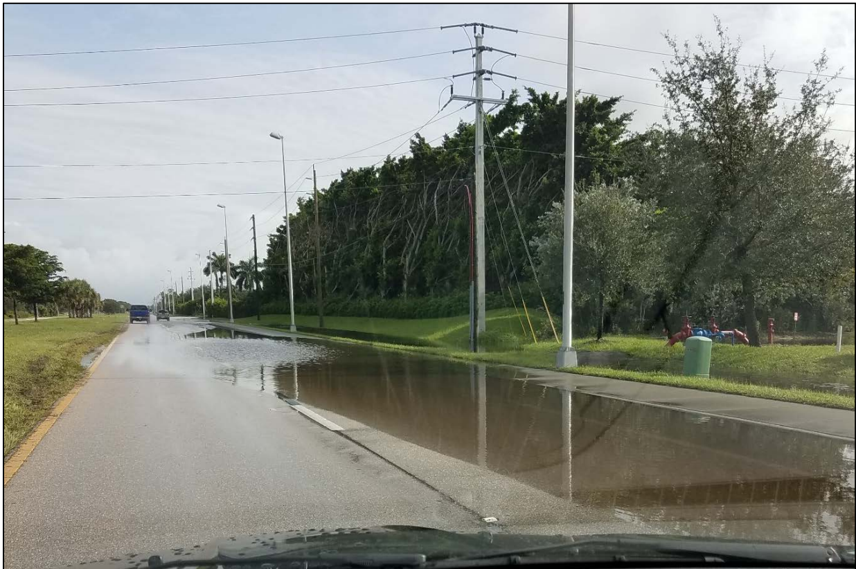
Figure 4-5: Three Oaks Parkway, Looking North (August 28, 2017)
