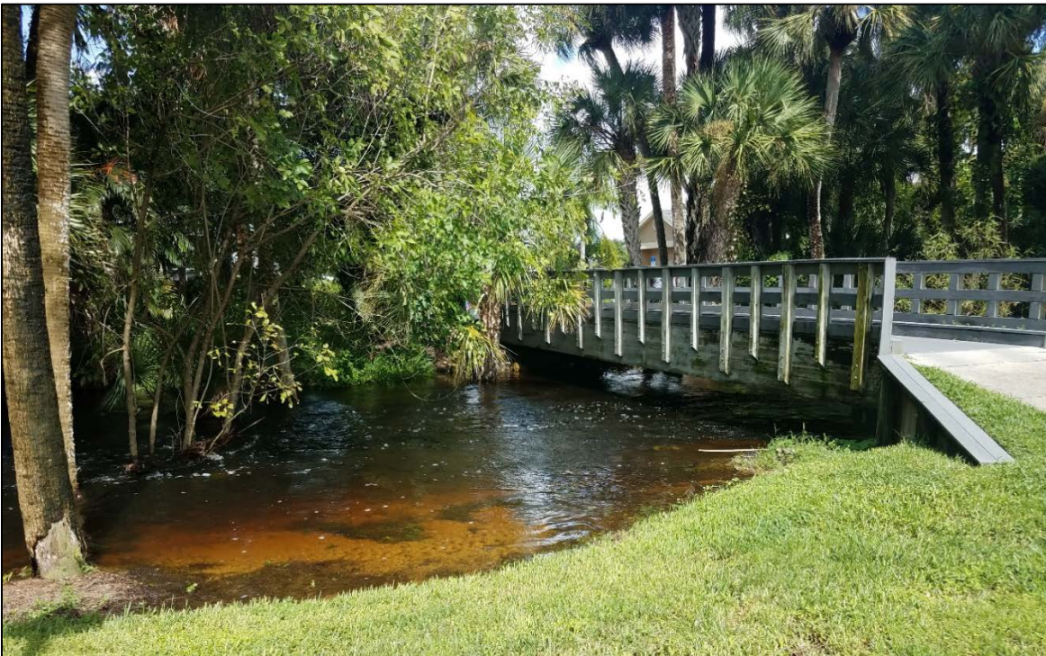
Figure 4-4: Estero River, North Branch (August 28, 2017)
