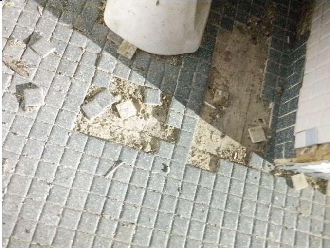
HM-BB: 1" Ceramic Tile/Grout/Mastic, Blue
