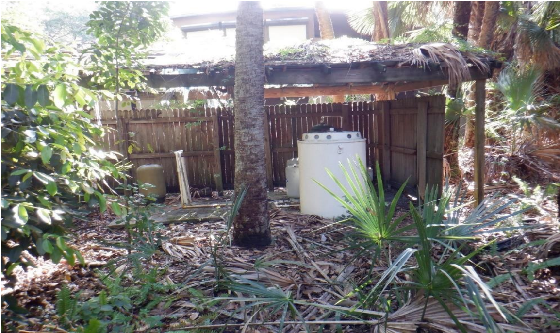
Photo 3: Structure 1 - 8661 Corkscrew Road 33928 – Woodshed for well and water equipment.
