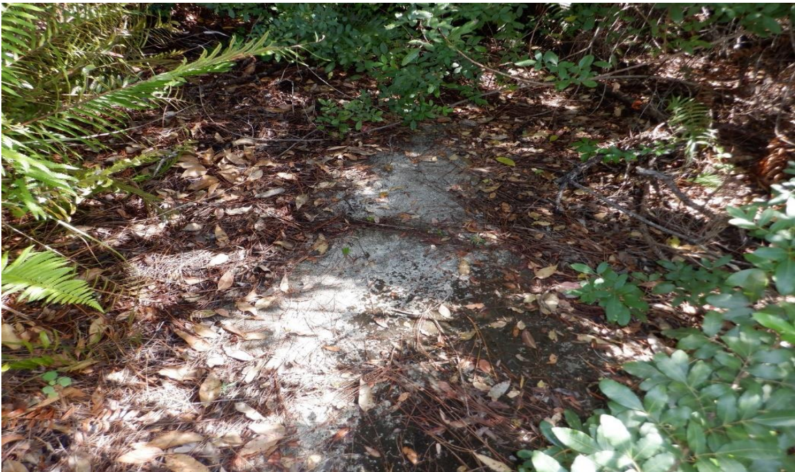
Photo 6: Structure 2 – Concrete slab approximately 100 ft 2
