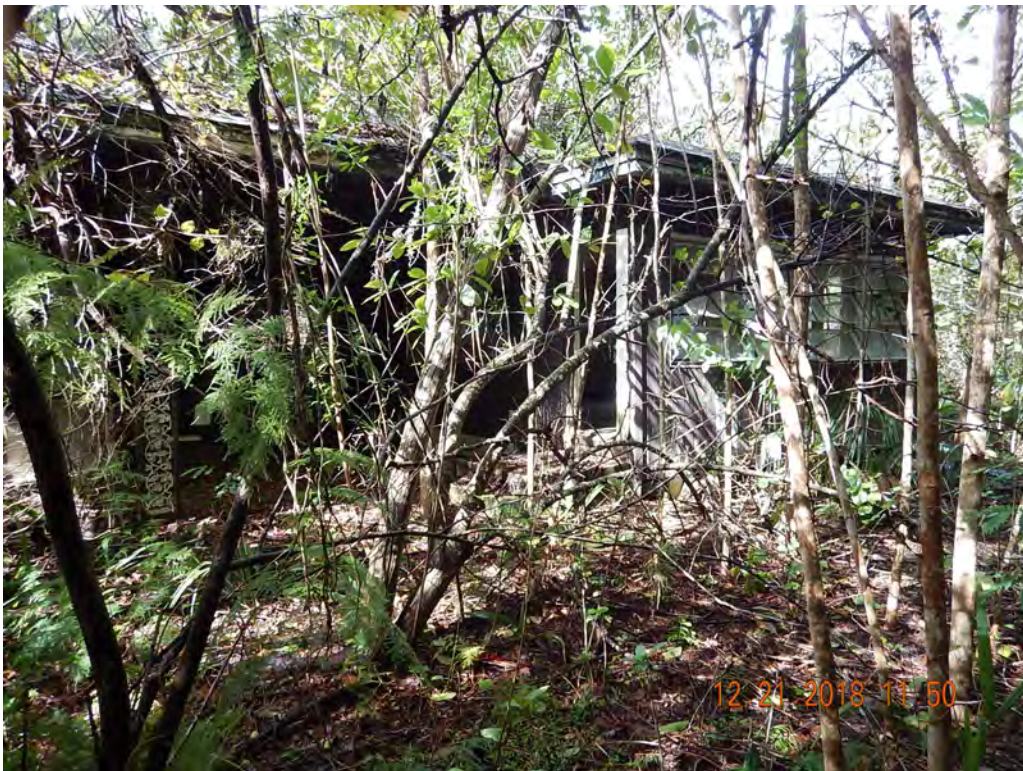
Photo #13 Looking NW at Structure 3
