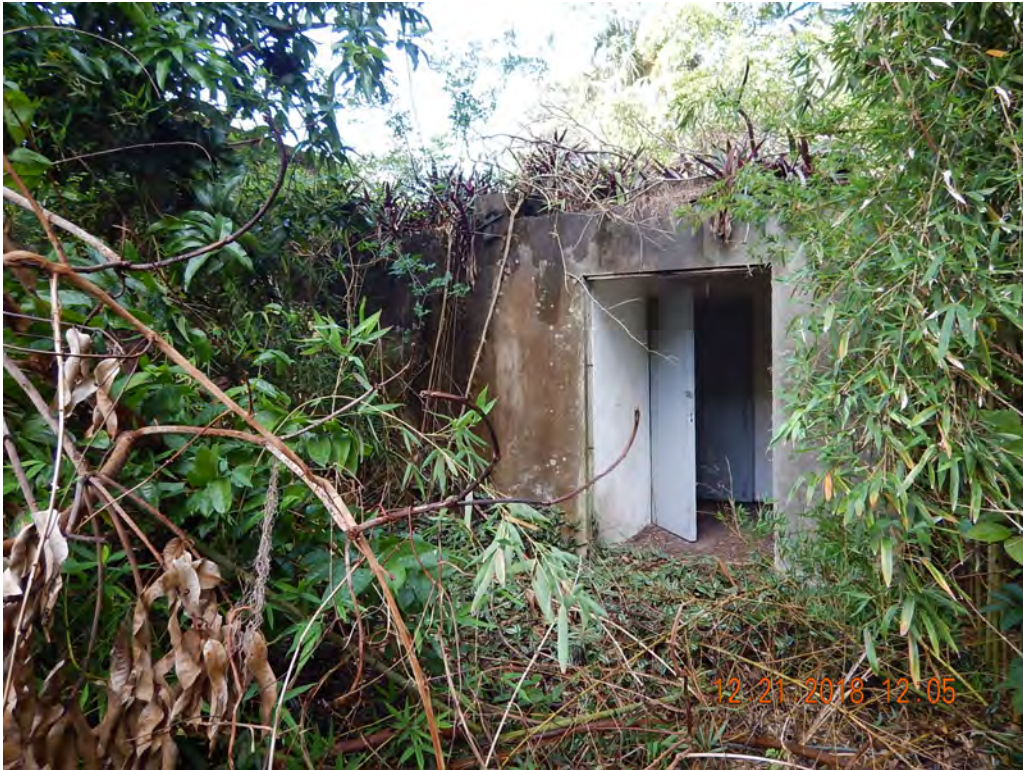
Photo #23 Looking W'ly at Structure 5
