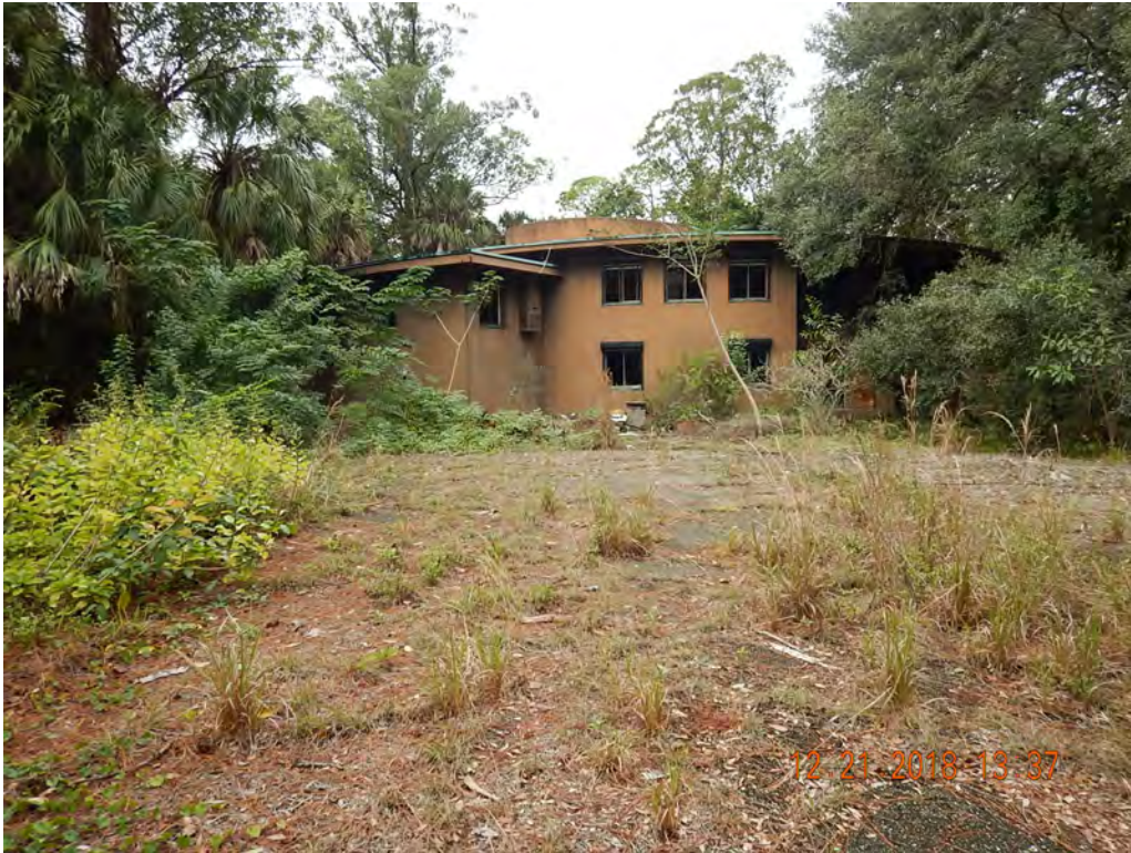
Photo #46 Looking West towards Structure 7
