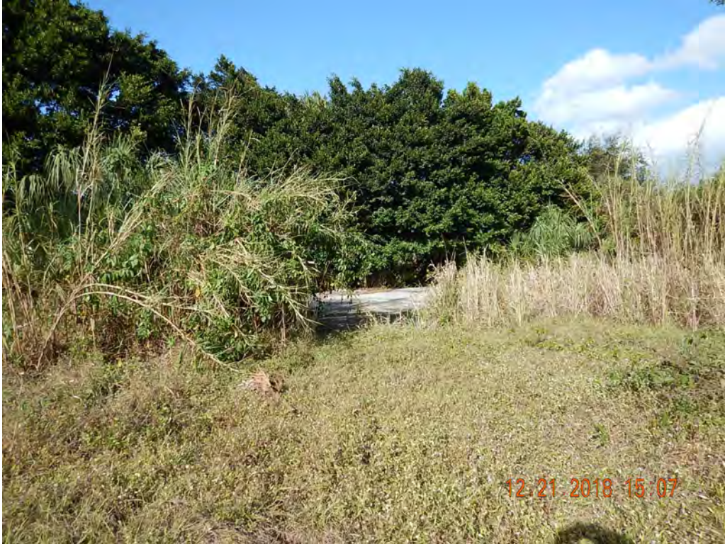
Photo #78 Looking NE at concrete slab
