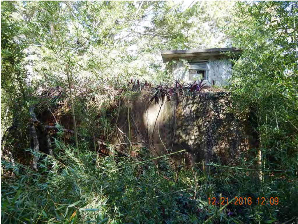
Photo #25 Looking NW at Structure 5
