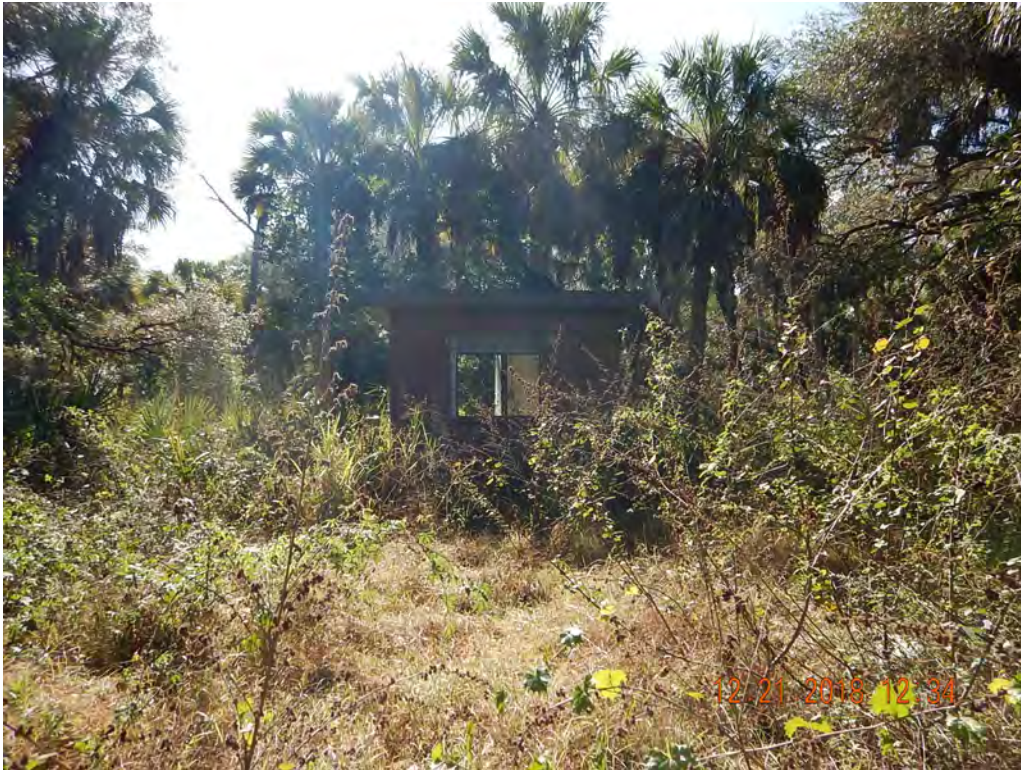
Photo #37 Looking SW at Structure 4
