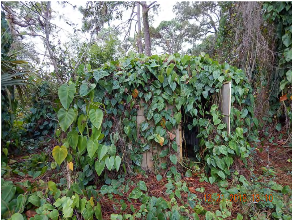
Photo #44 Alum Shed SW of Structure 9
