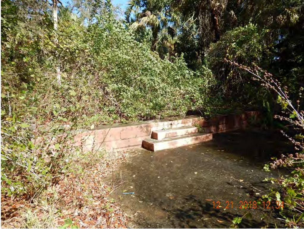
Photo #36 Looking SW at Structure 2
