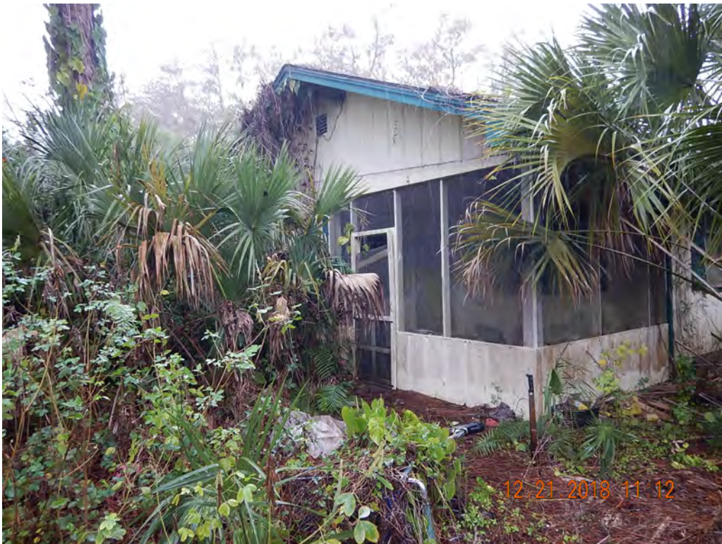
Photo #8 Looking NE at Structure 9
