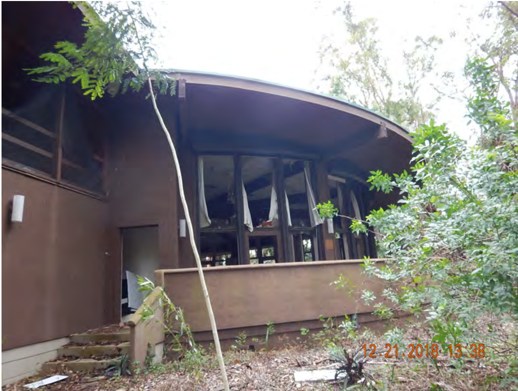
Photo #48 Looking West towards Structure 7
