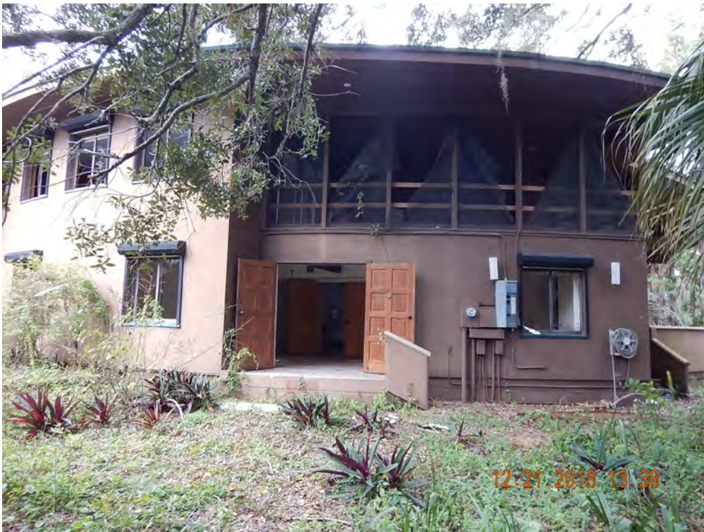
Photo #47 Looking West towards Structure 7
