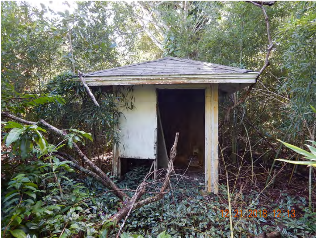
Photo #28 Looking SE at Structure 6
