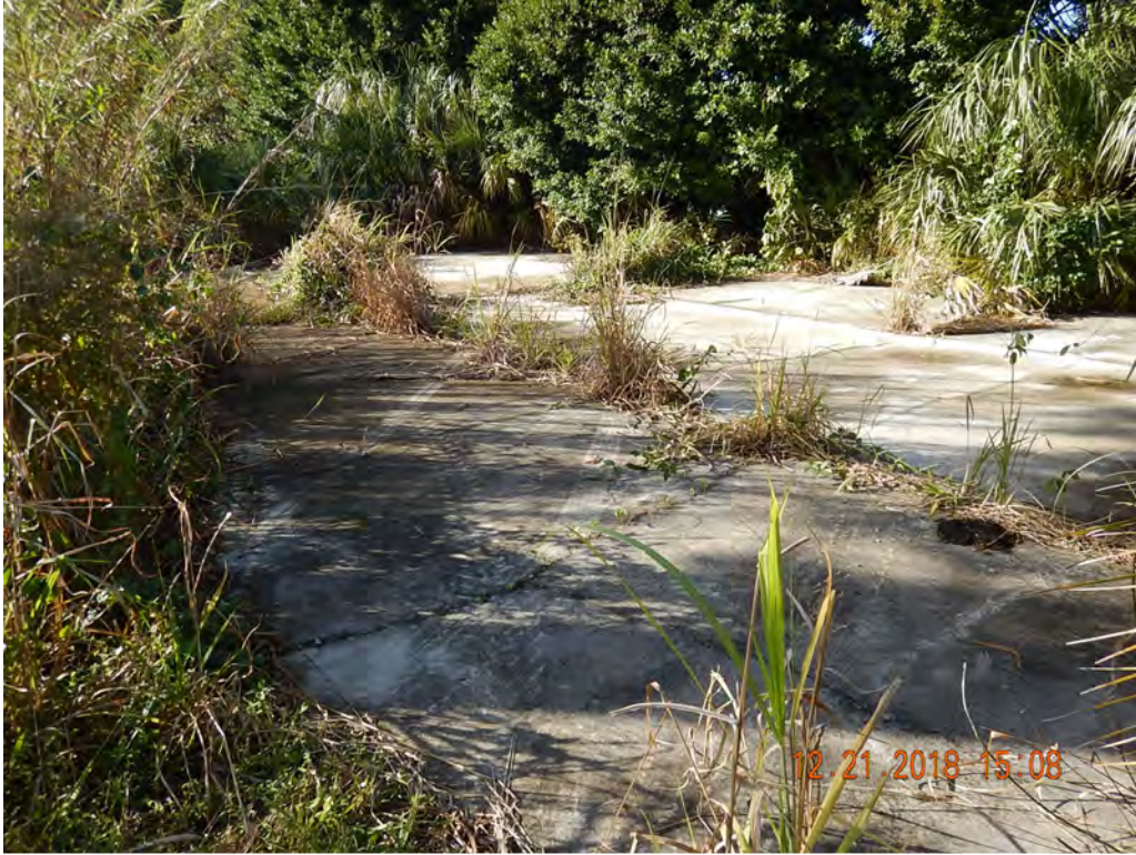
Photo #80 Looking NW at concrete slab
