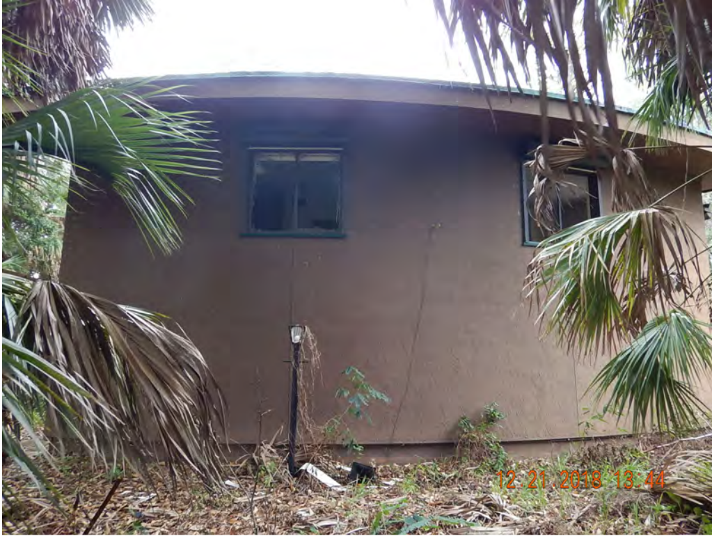
Photo #56 Looking NE at Structure 7
