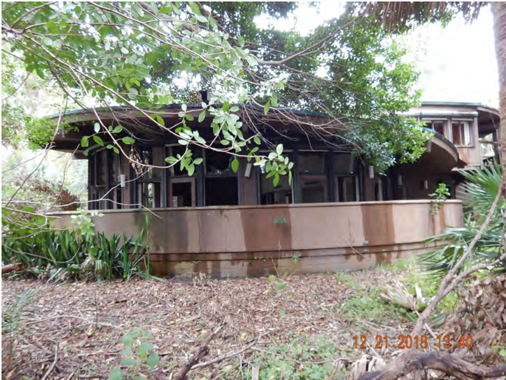
Photo #51 Looking West at Structure 7
