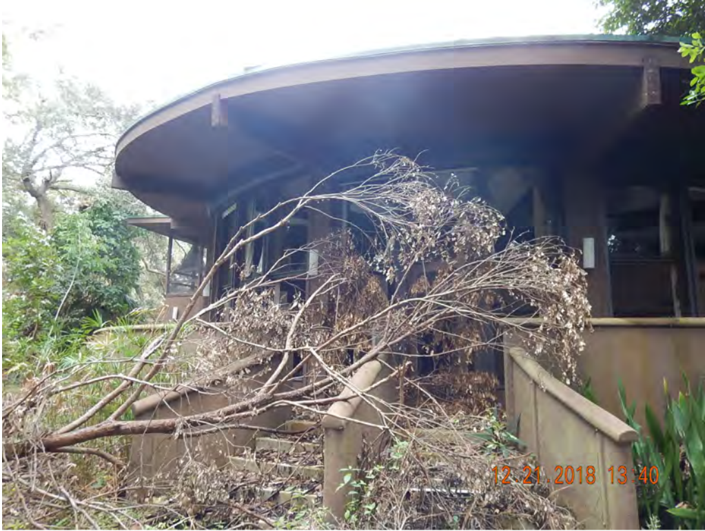
Photo #50 Looking SE at Structure 7
