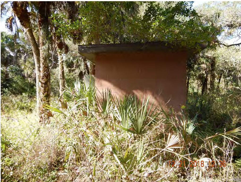
Photo #38 Looking NW at Structure 4
