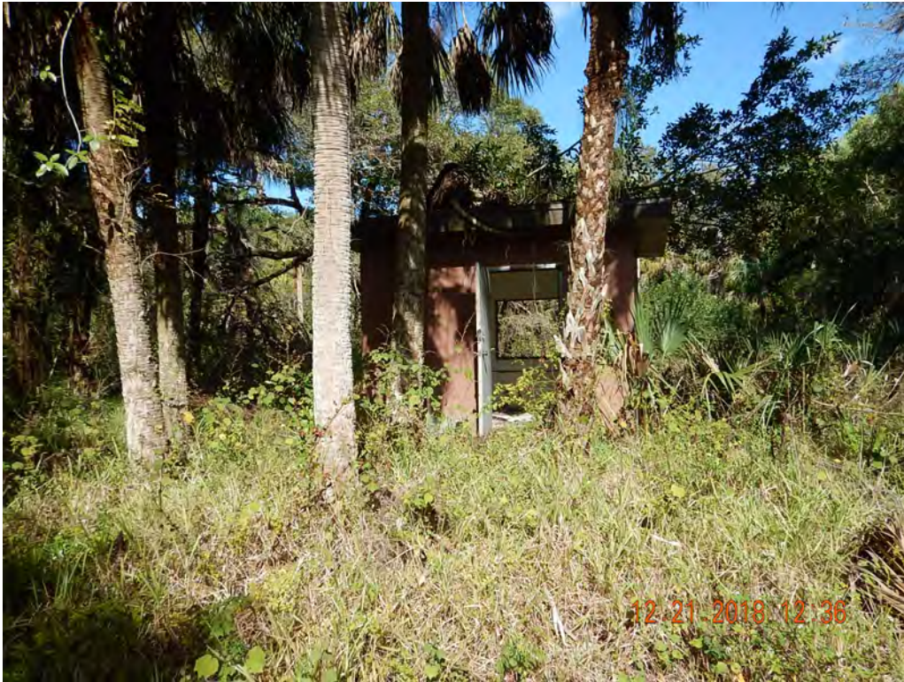
Photo #39 Looking NE at Structure 4
