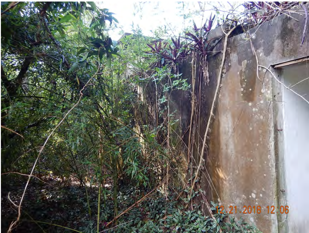
Photo #24 Looking W'ly at Structure 5
