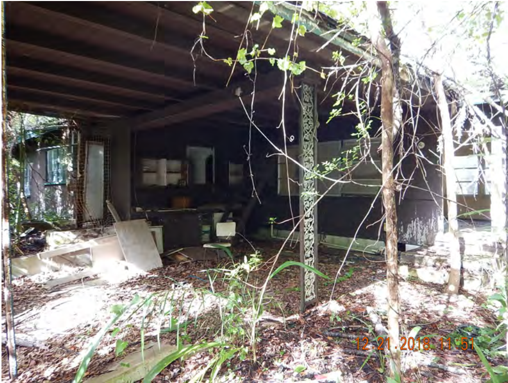
Photo #14 Looking NW at carport Structure 3
