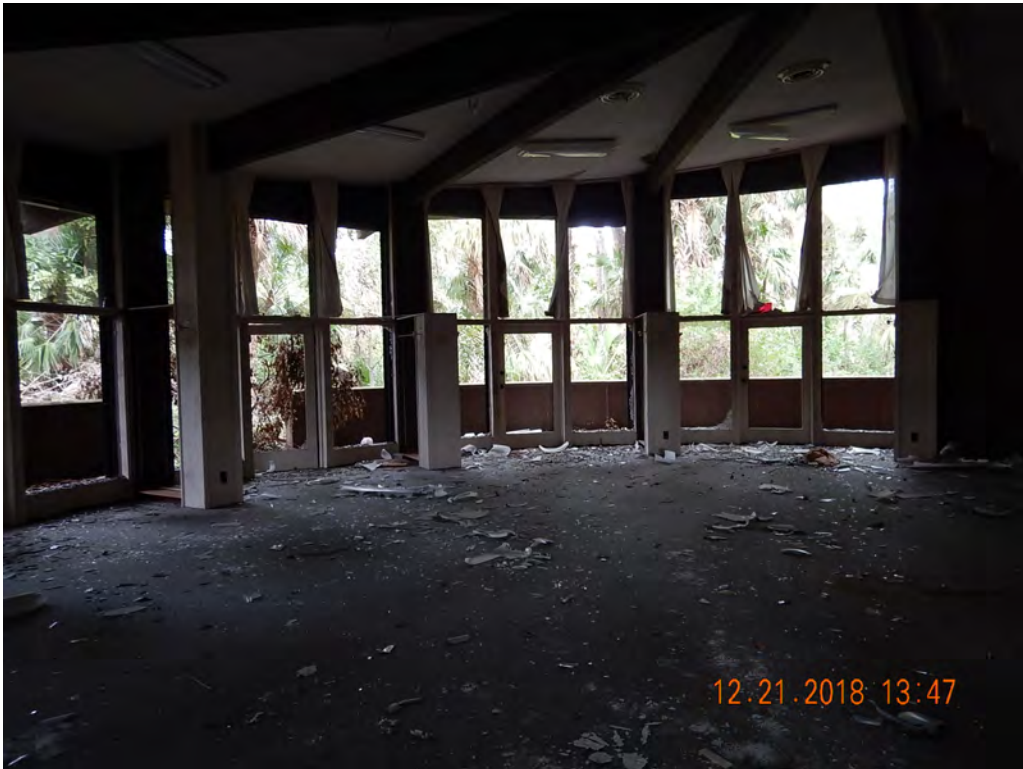
Photo #57 Looking East inside Structure 7
