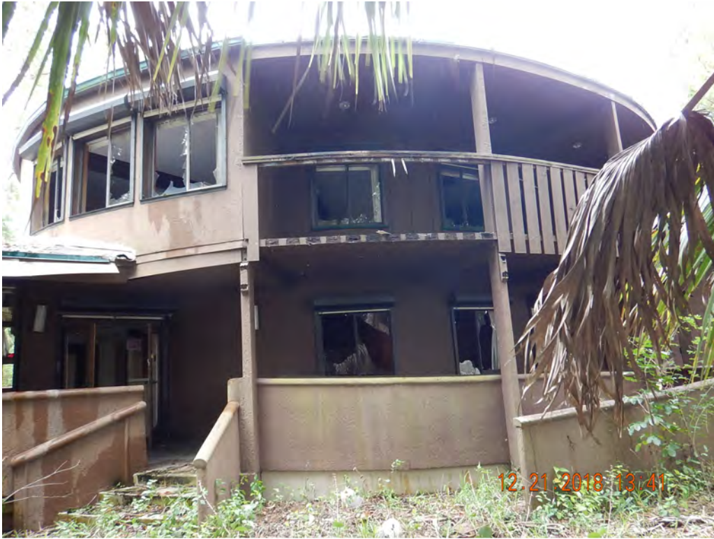
Photo #54 Looking NW at Structure 7
