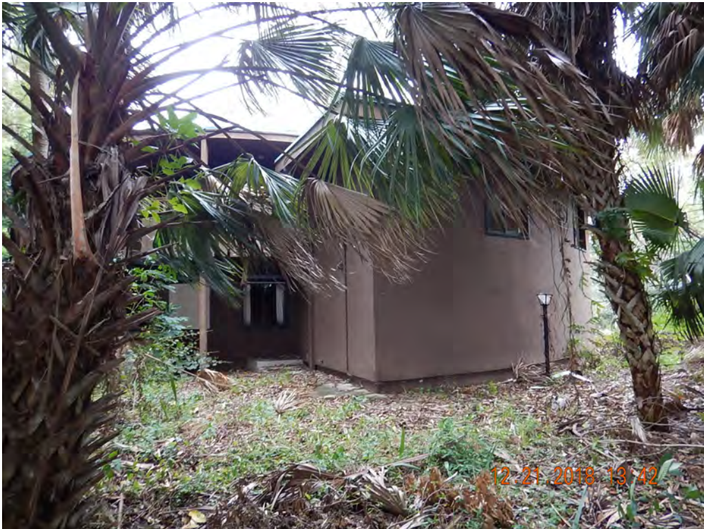
Photo #55 Looking North at Structure 7
