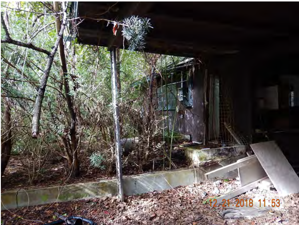
Photo #17 Looking NW at south entrance Structure 3
