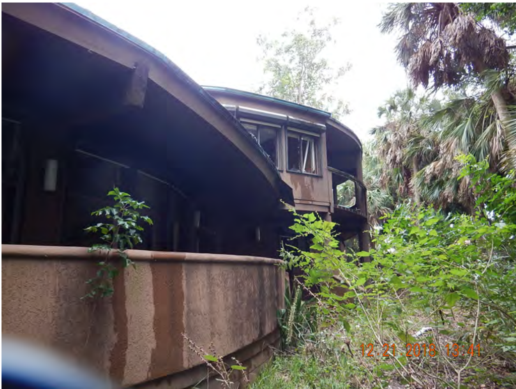
Photo #53 Looking SE at Structure 7
