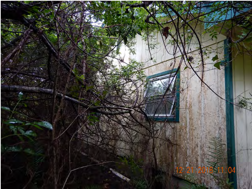
Photo #3 Looking SE at Structure 9
