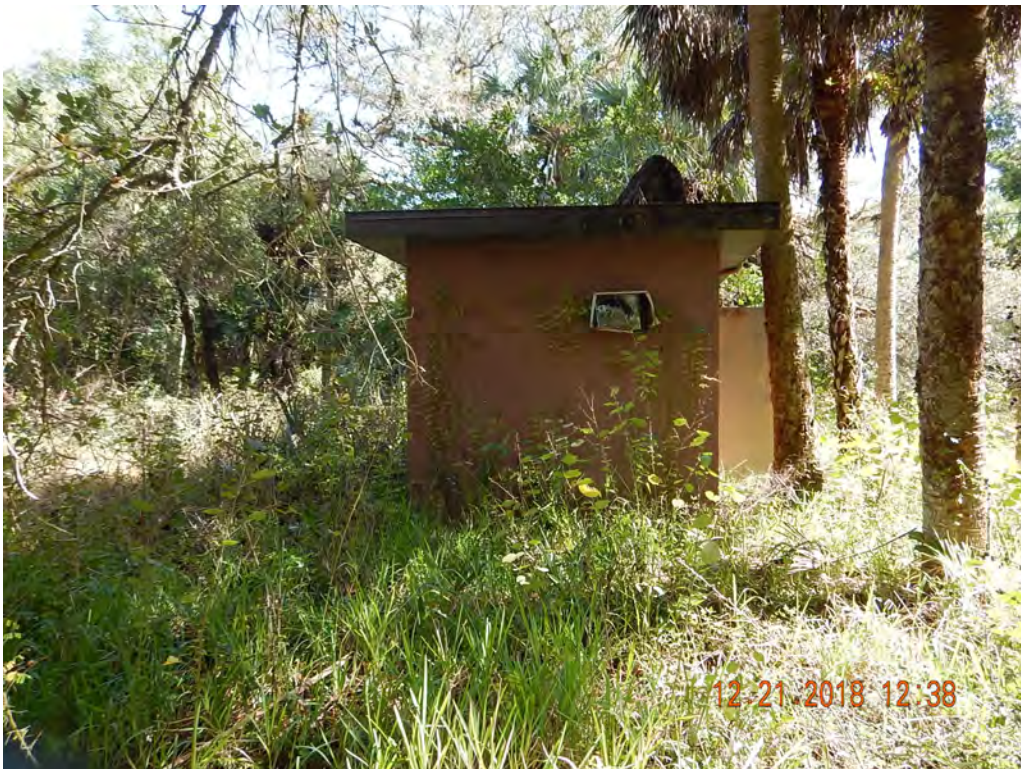
Photo #40 Looking SW at Structure 4
