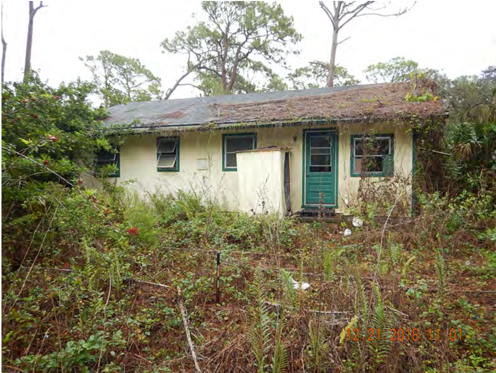
Photo #2 Looking NE at Structure 9
