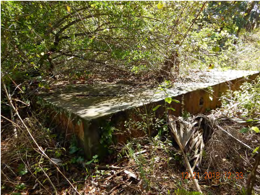
Photo #35 Looking SE at Structure 2
