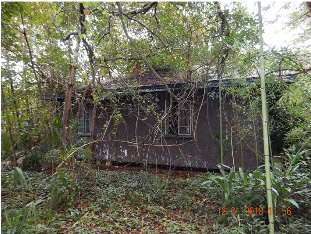
Photo #19 Looking NE at Structure 3
