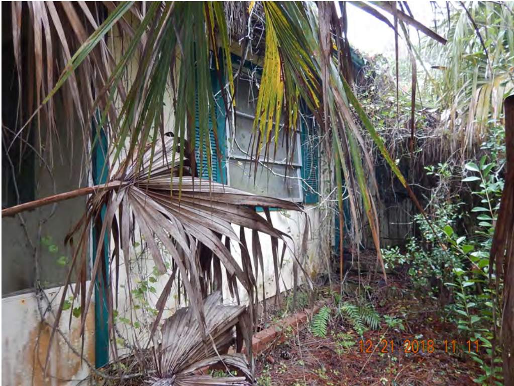
Photo #6 Looking NE at Structure 9
