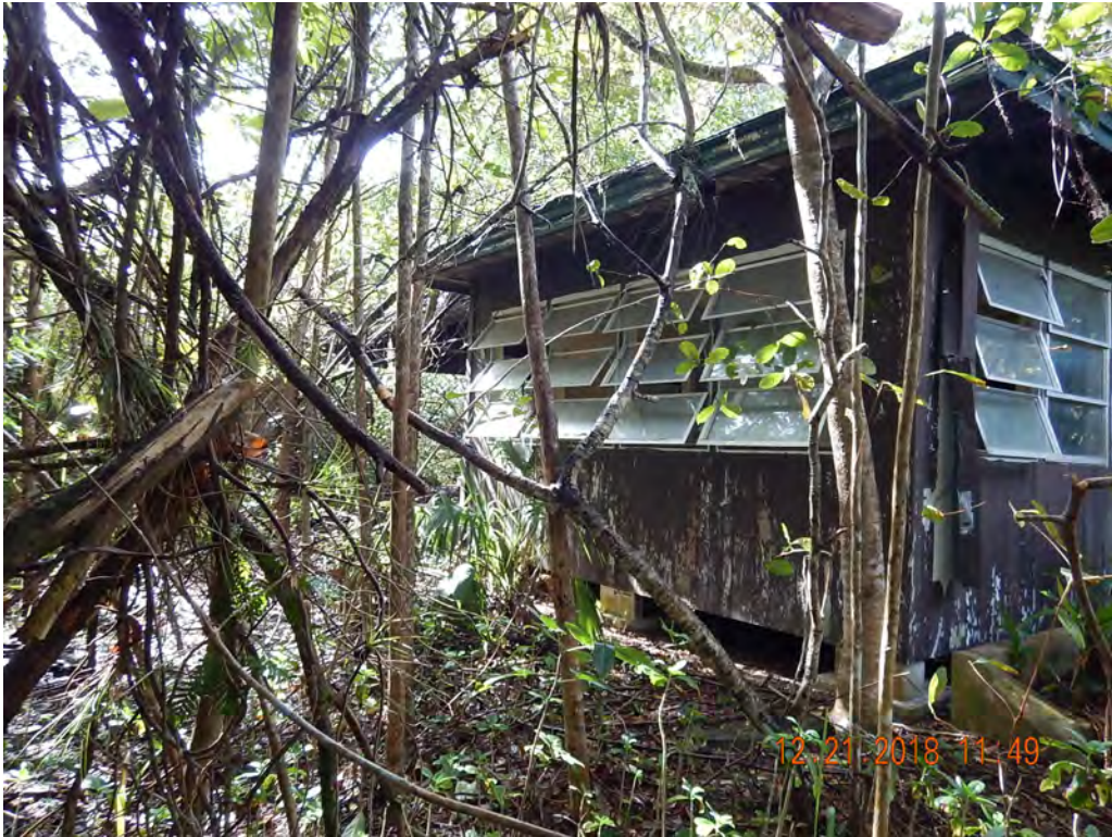
Photo #12 Looking SW at Structure 3
