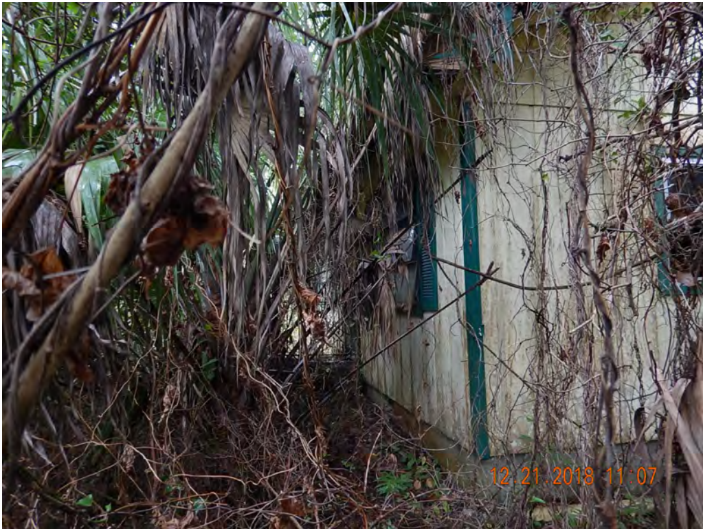
Photo #5 Looking SW at Structure 9
