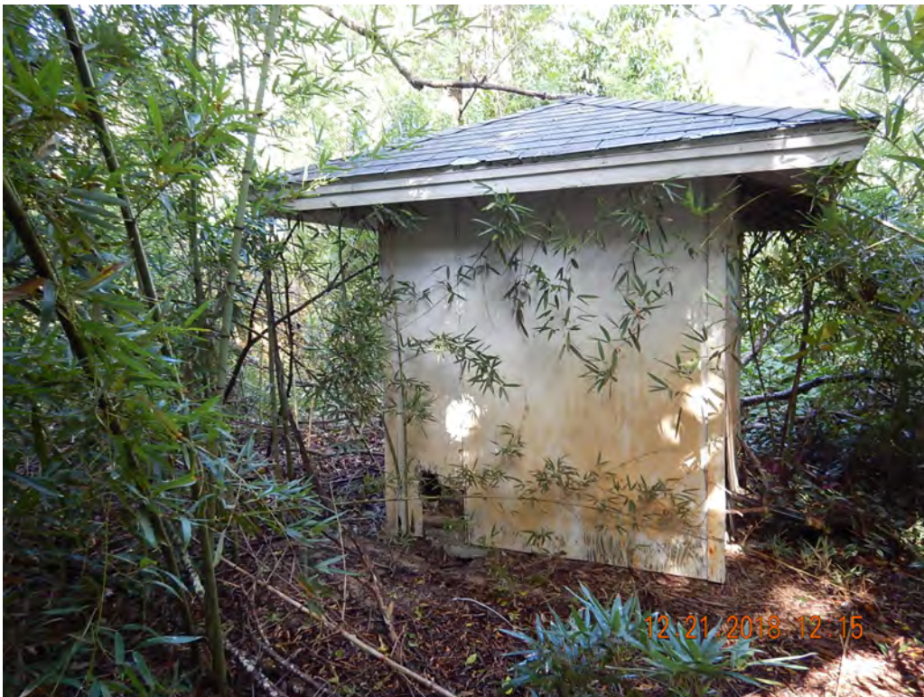
Photo #29 Looking NE at Structure 6
