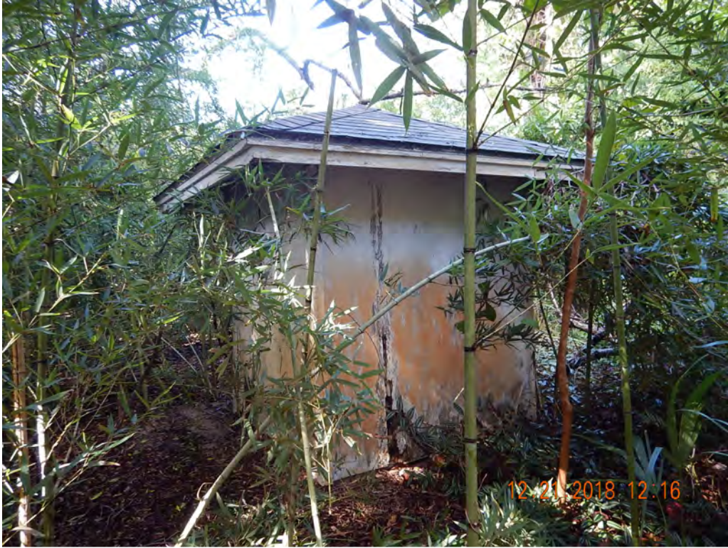
Photo #30 Looking E'ly at Structure 6
