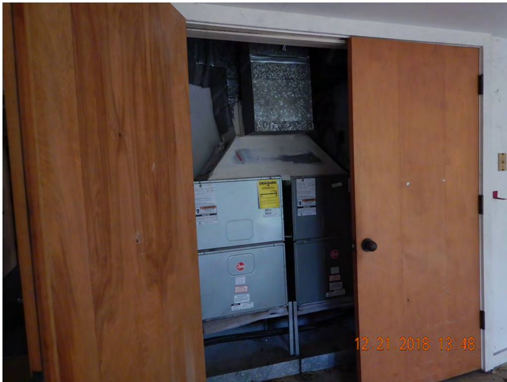
Photo #59 Looking NW inside Structure 7
