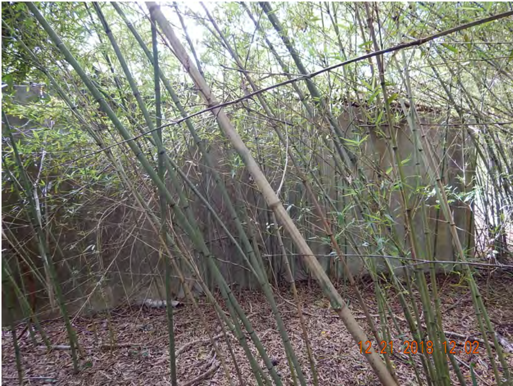
Photo #22 Looking SW at Structure 5
