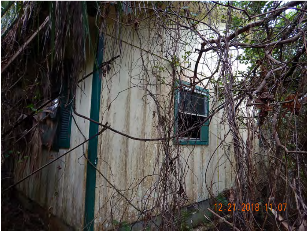
Photo #4 Looking SW at Structure 9
