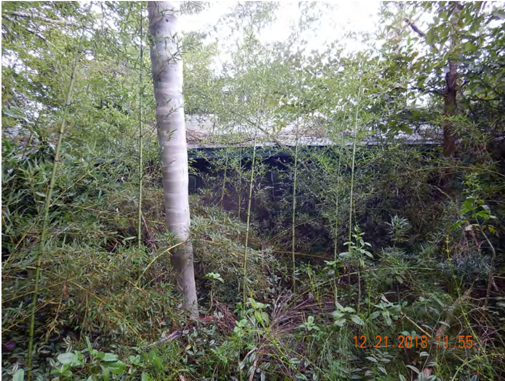
Photo #18 Looking North at Structure 3
