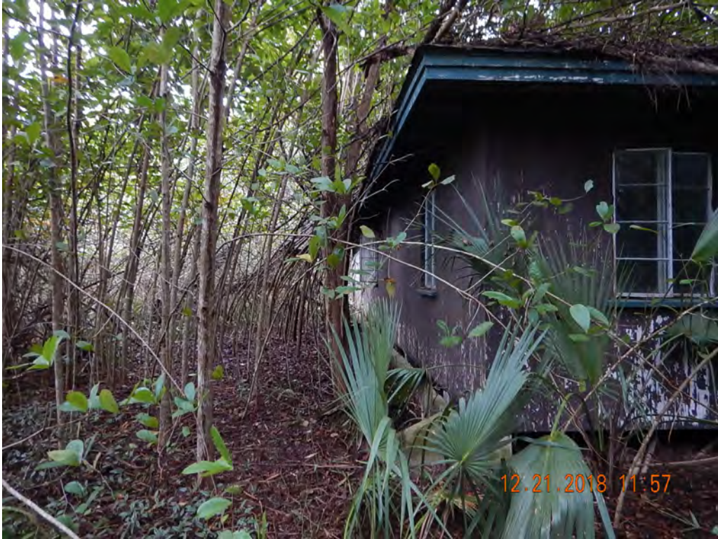
Photo #20 Looking West at Structure 3
