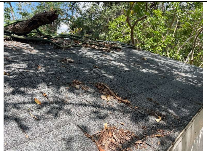
HM-P: Asphalt Shingle/Felt, Black
