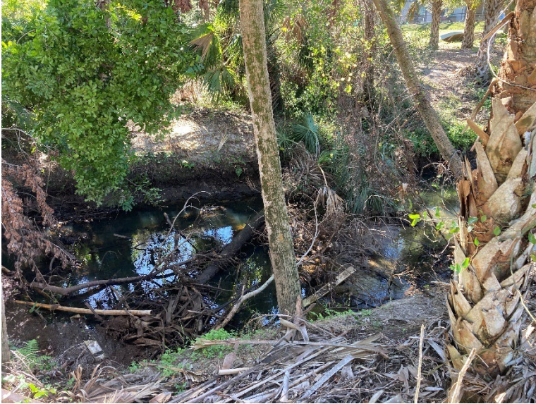
Palm tree and debris behind 9168 Estero River Circle looking from Villages at Country Creek side.
