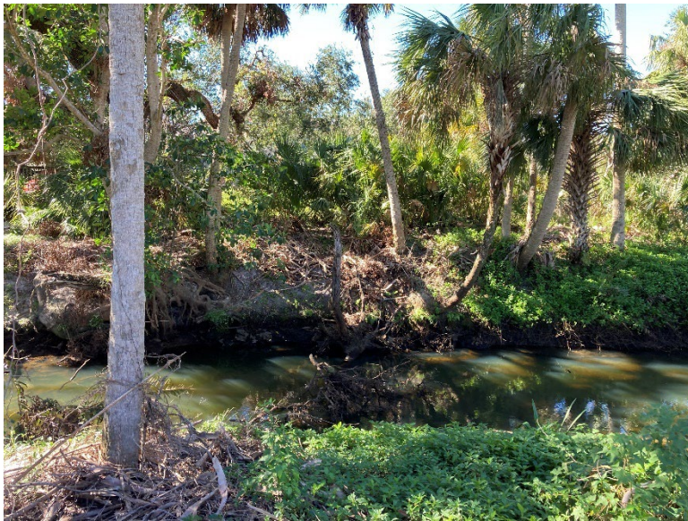
Tree limbs in South Branch just downstream of 9174 Estero River Circle looking from Villages at Country Creek side.
