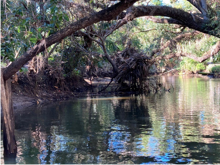
Tree limbs and debris at approximately 9264 Estero River Circle
