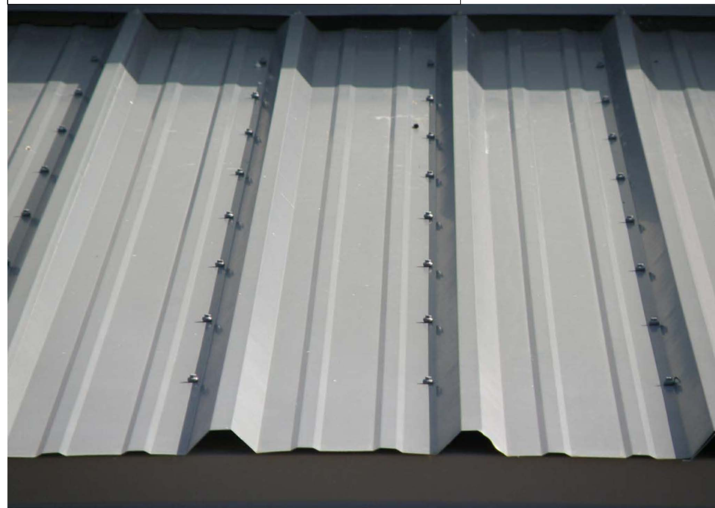
METAL ROOF FOR AWNING
