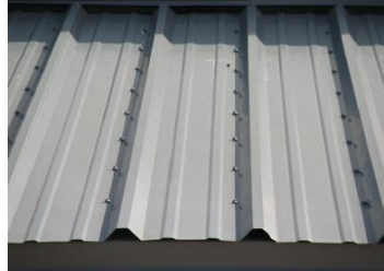
METAL ROOF FOR AWNING
